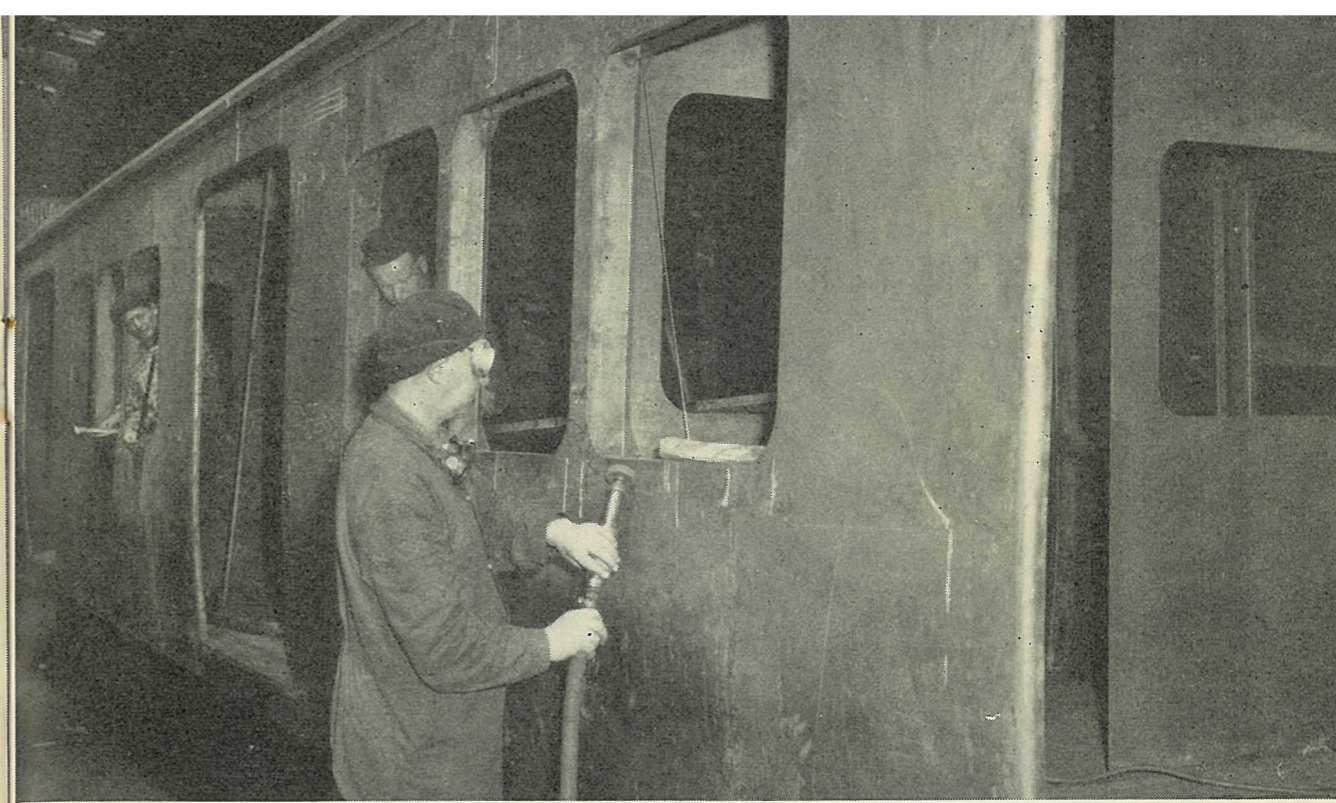
FINISHING OFF WELDED SIDES OF A "HARRIS TRAIN" TRAILER CARRIAGE
